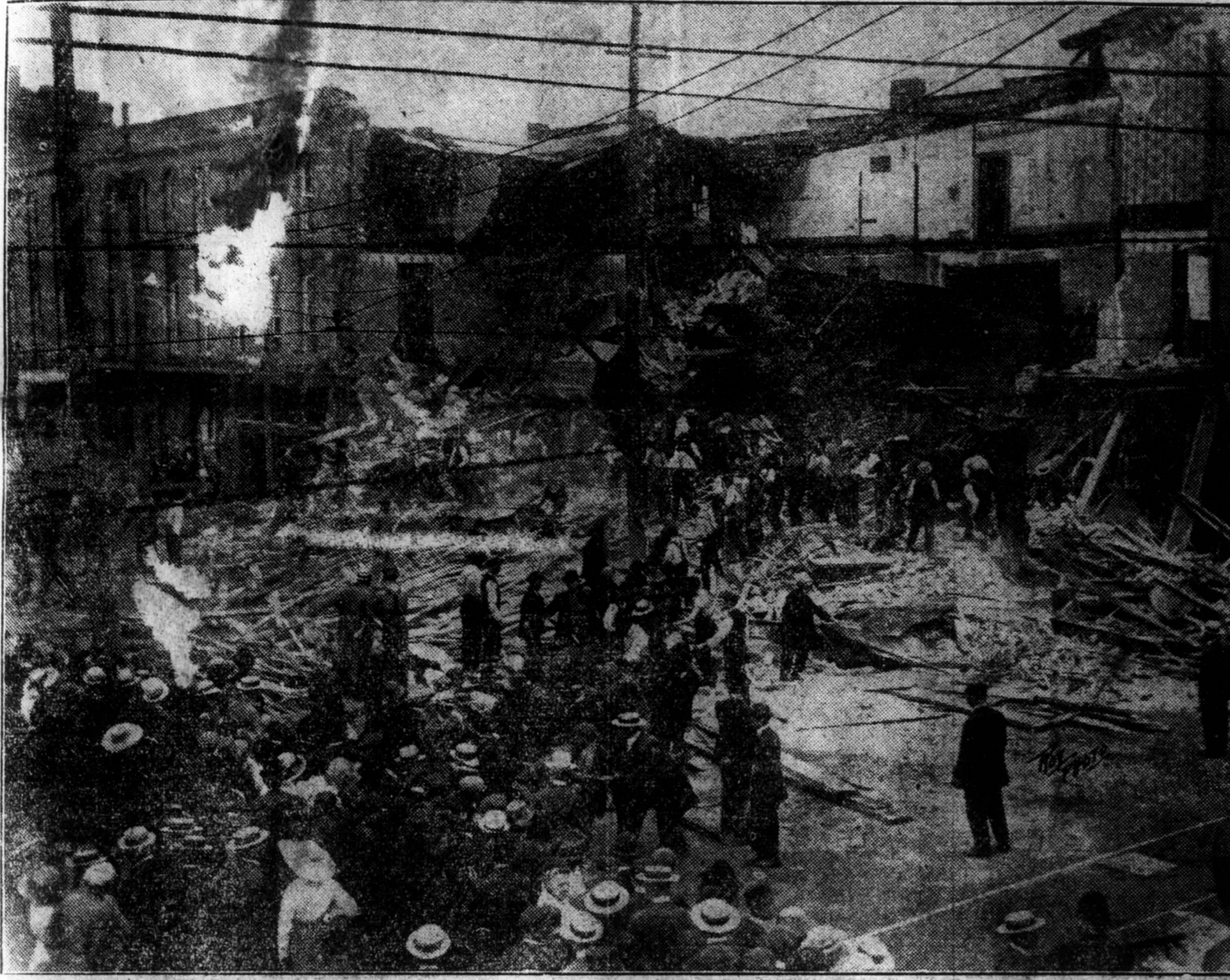
Photo of Wreckage of Turnbull's Store Which Collapsed
