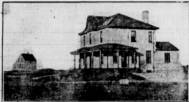
Superintendent's Residence, Nursery Station at Indian Head, 1905
