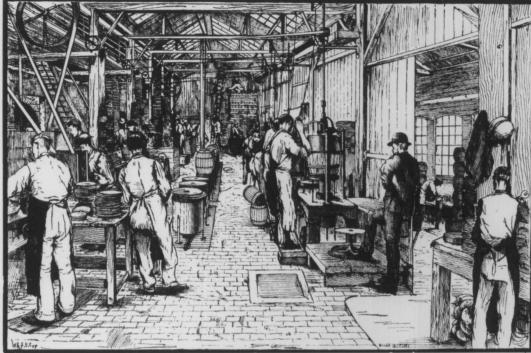
the iron hoops, forced on by the hydraulic presses, are knocked away. Some thousands of casks, of various sizes, are manufactured weekly. A stranger would
