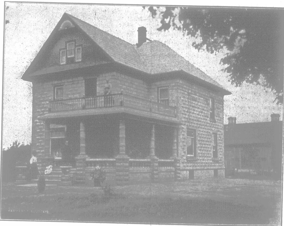
New residence of Wm. Butler, Lambton Co., Ont. A most completely equipped house, with excellent situation.
