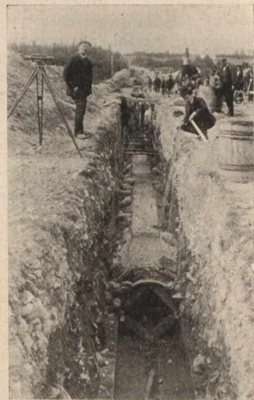
Concrete Conduit in Trench.
