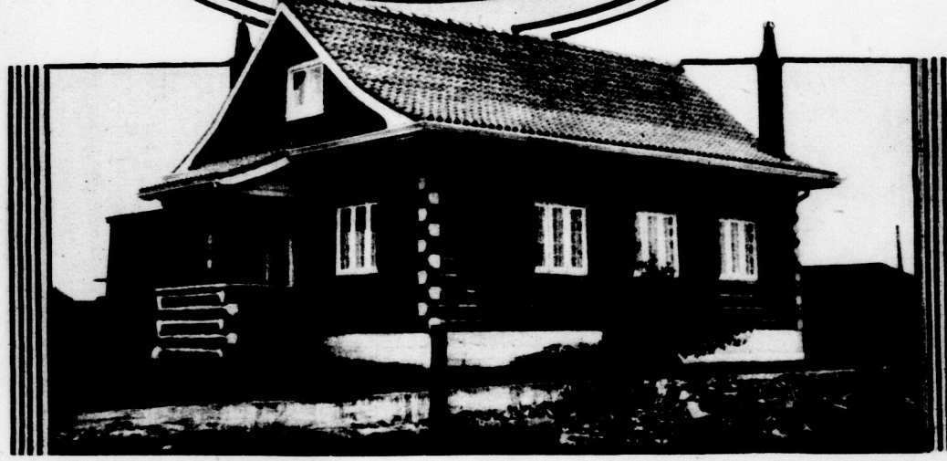
A little bungalow at Mimico, on the outskirts of Toronto, is built and roofed entirely of sewer pipe of different sizes
