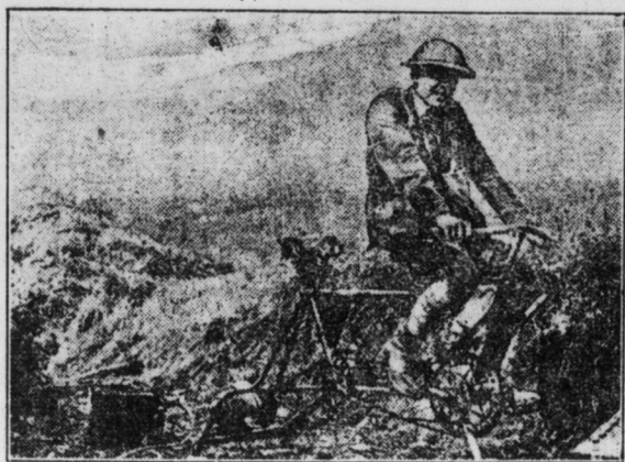
Taken From The Enemy—A British soldier demonstrating a device used by the Germans for generating electricity to operate their wireless apparatus in the trenches.
