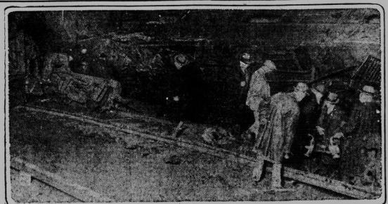
Investigations are being made of the wreck of the second section of the Pennsylvania railroad's New York-Atlantic City flyer at Delair, N. J., in which several were killed and more than 40 injured. A split rail on a curve is believed to have been responsible. Two views of the wreckage.
