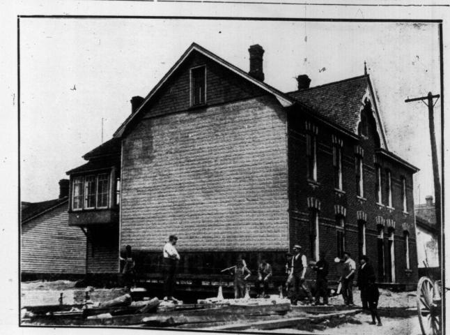
SUCCESSFUL FIRST ATTEMPT OF AMATEURS. A 3-storey brick house on DeGrassi-street being moved to a new site. The work was successfully performed by four novices in the house-moving art,
