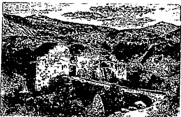
BRIDGE AND GATEWAY AT BANIAS, CAESAREA-PHILIPPI
