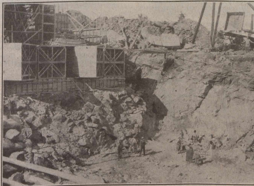
EXCAVATION FOR POWER-HOUSE
