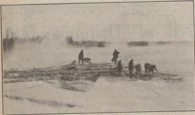
PLACING COFFERDAM CRIBS IN JANUARY
