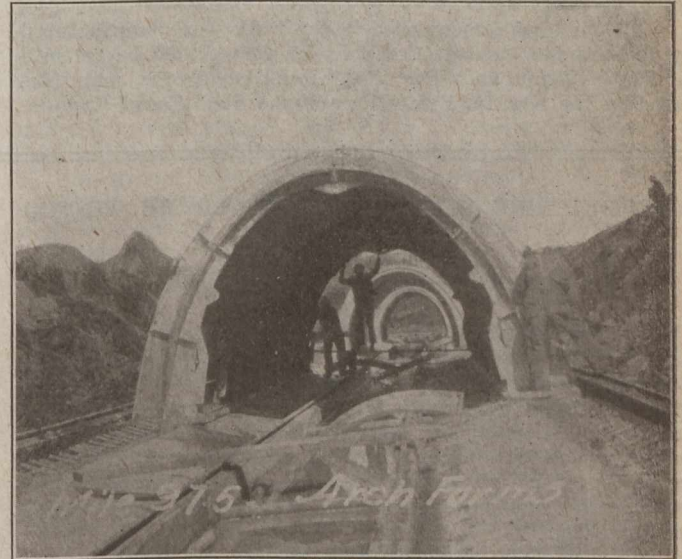
ERECTING STEEL ARCH FORMS FOR 10 FT. 9 IN. BY 9 FT. AQUEDUCT
