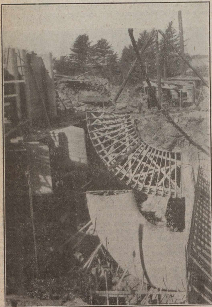
PLACING FORMS FOR DRAFT TUBES
