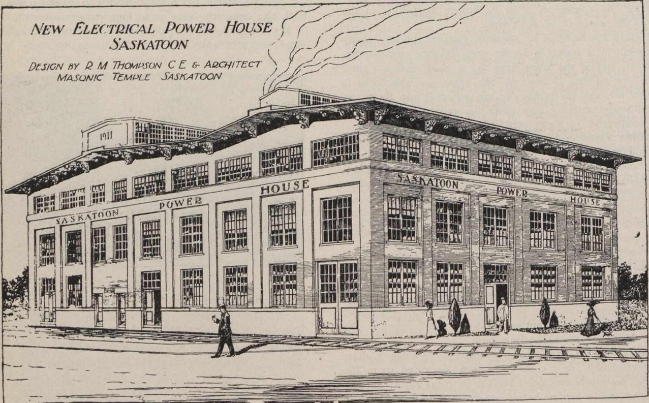
The construction is of steel, brick, and concrete, and is fireproof. The dimensions are 85 by 154 feet, and the walls are 42 feet high; the construction is of the most modern for
