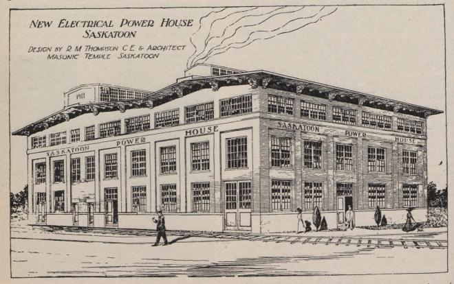
The construction is of steel, brick, and concrete, and is fireproof. The dimensions are 85 by 154 feet, and the walls are 42 feet high; the construction is of the most modern for in the boiler-room, the boiler equipment consists of three double cylinder water tube Babcock and Wilcox boilers, each of a rated capacity of 500 horse-power, but used in conjunc-
