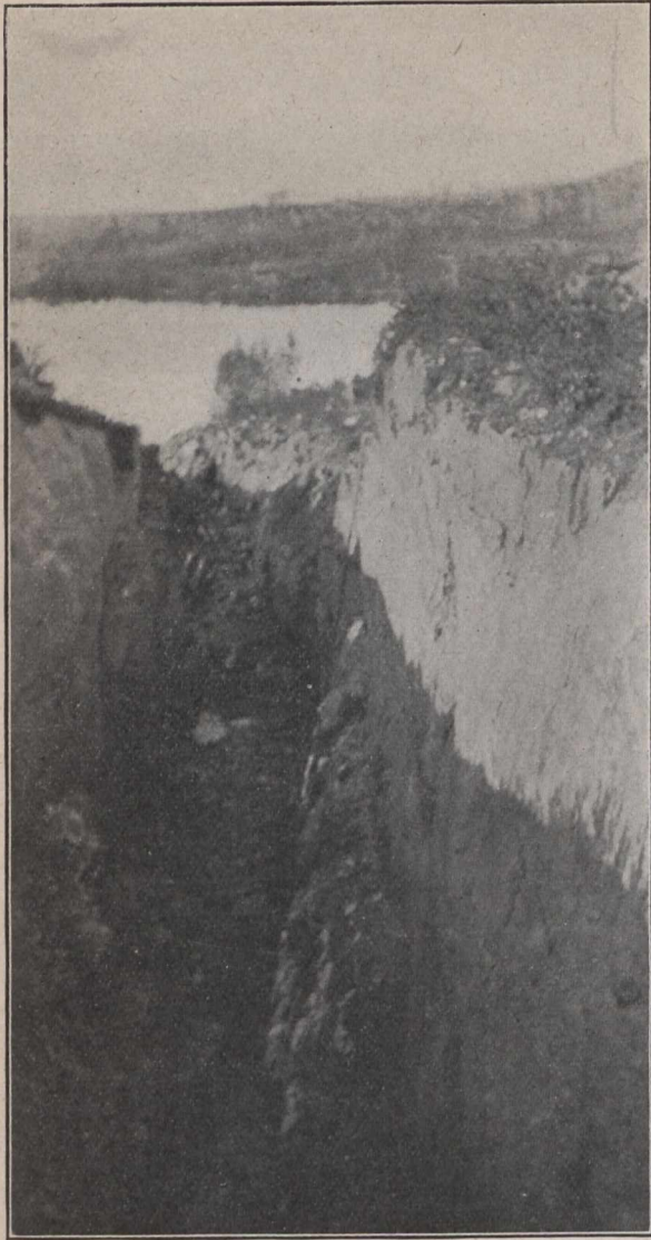
Open Cut running north from the shore of Coture Lake.
