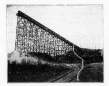
Figure 2 shows the conveyor, which, as can be seen, consists of a "Century" belt running on special troughing idlers. It is known as the "Jeffrey Century" type, which means a specially high grade rubber belt, covered with an extra coat of rubber, which is particularly designed for withstanding wear and tear of the material handled.
