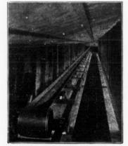
In this point the material is discharged at the terminal; special tripping devices are provided where it is necessary to discharge material at intermediate points. This style of carrier is also designed for carrying crushed stone, gravel, etc.
