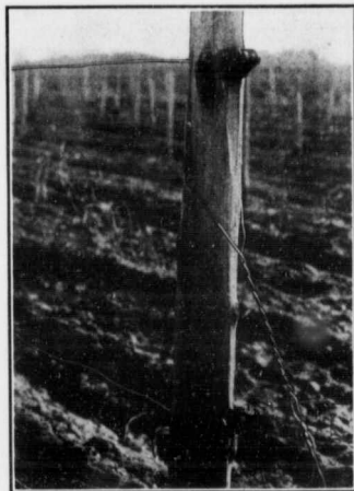
A common patent used for taking up the slack in the wire.
