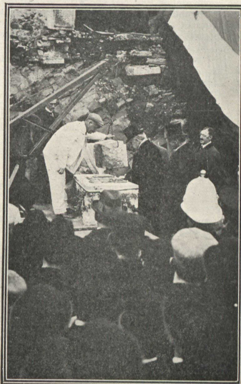
LAYING THE POST-OFFICE CORNER-STONE. The Premier Well and Truly Lays the Corner-stone of the New Quebec Post-Office.
