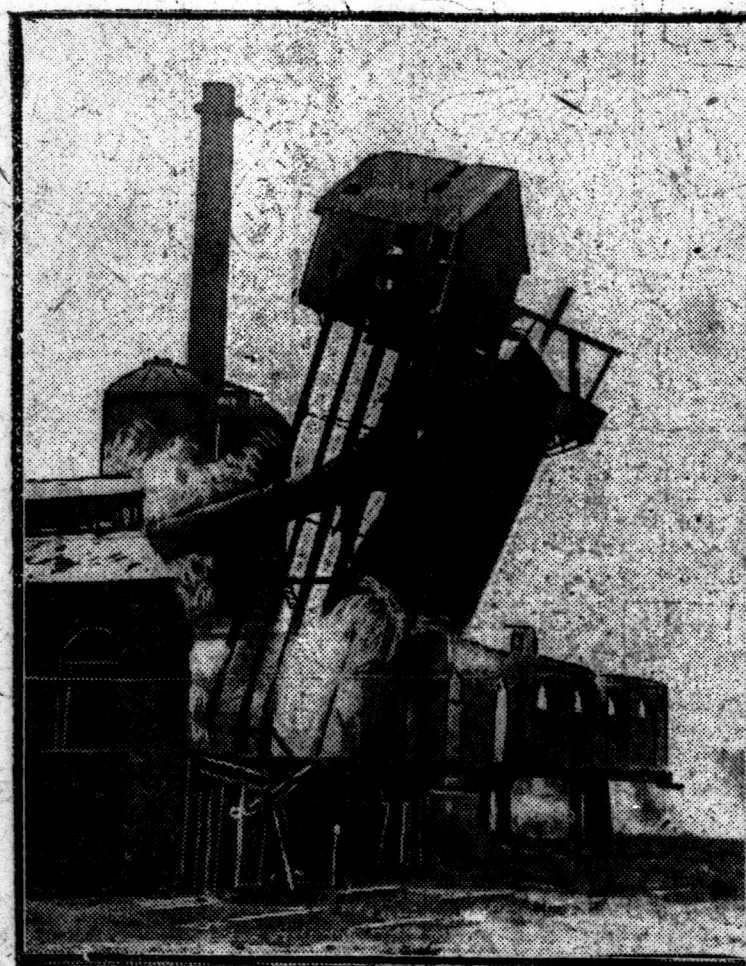
The ordinary method of wrecking buildings being considered too slow, the Pettstown Iron Works used dynamite to clear away their old blast furnaces.
