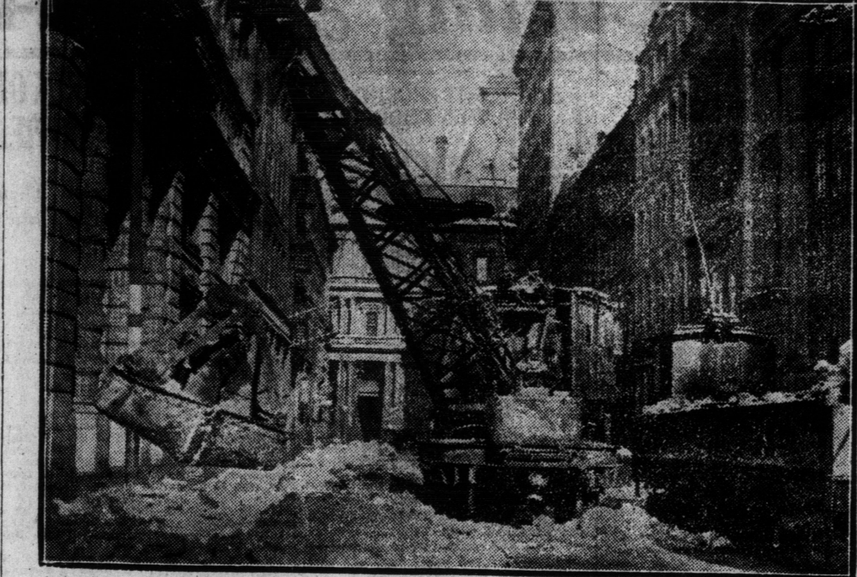
Hand shovellers were put to shame when this electric shovel came to the fore and took a hand at removing the snow from Federal street, Boston, recently. Pile after pile of snow and ice was gathered up and carried off in electric cars in a jiffy.
