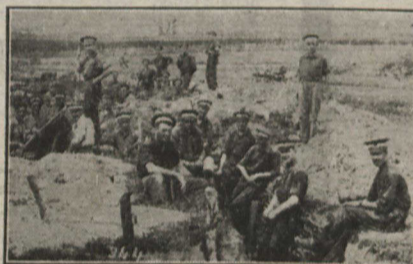
Cadet Company on the Entrenching Area
