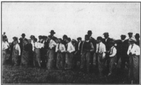
Preparation for the Start.
