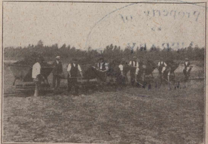
FIG. 8—FILLING WAGONS WITH DRY SLUDGE
