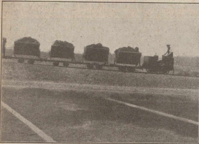
FIG. 7—FIVE TIP WAGONS DRAWN BY ELECTRIC BATTERY LOCOMOTIVE
