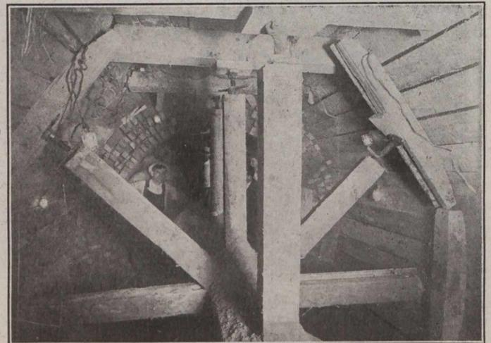
Fig. 5.—Illustrating the Needle-beam Method of Supporting the Sheeting as the Tunnel Progresses.
