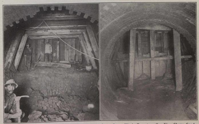
Fig. 1.—Tunnel Headings 80 Feet Apart in the Keele Street Sewer Work, Toronto. One View Shows Good Working Clay and the Other a Heavy Water Seepage Requiring 12 to 18 lbs. of Compressed Air.
