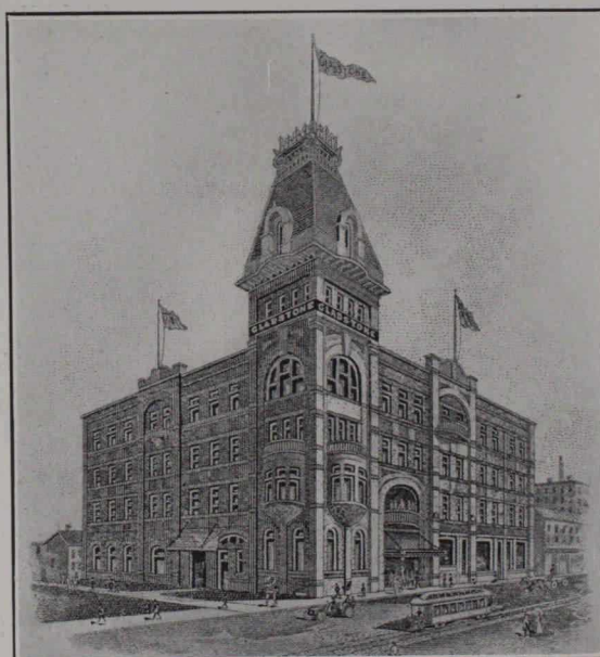
The Gladstone Hotel, 1204 Queen Street, West.
