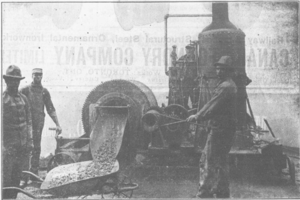
RANSOME MIXER COMPLETE WITH ENGINE AND BOILER, ALSO SHOWING OUR SPECIAL HOISTING ATTACHMENT.
