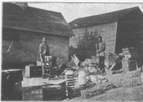
A Preliminary Stage in the Construction of a Cement Block Silo
