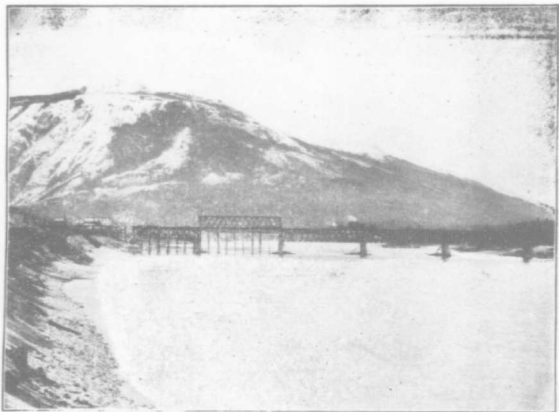
FIRST RAILWAY BRIDGE ACROSS COLUMBIA RIVER, REVELSTOKE
