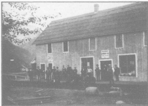
MUNDY LUMBER CO'S STORE AND OFFICES, THREE VALLEY.
