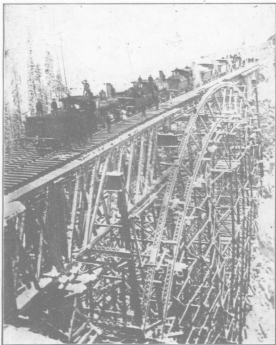
TEST OF STONEY CREEK BRIDGE, on completion of construction.
