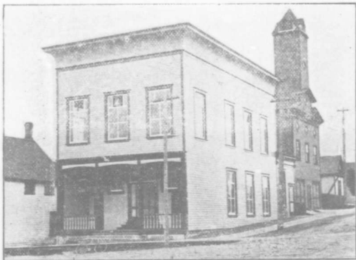
CITY HALL AND No. 2 FIRE HALL.
