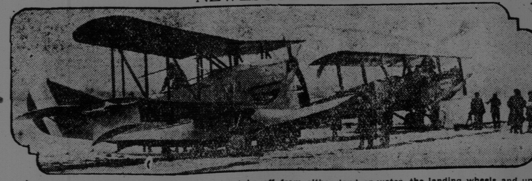
They are amphibian and can land on or take off from either land or water, the landing wheels and under-carriage being raised and packed into the pontoon, or brought from the pontoon into landing position, in a few seconds, at the will of the pilot while in flight. They are known as the Leoning planes.
