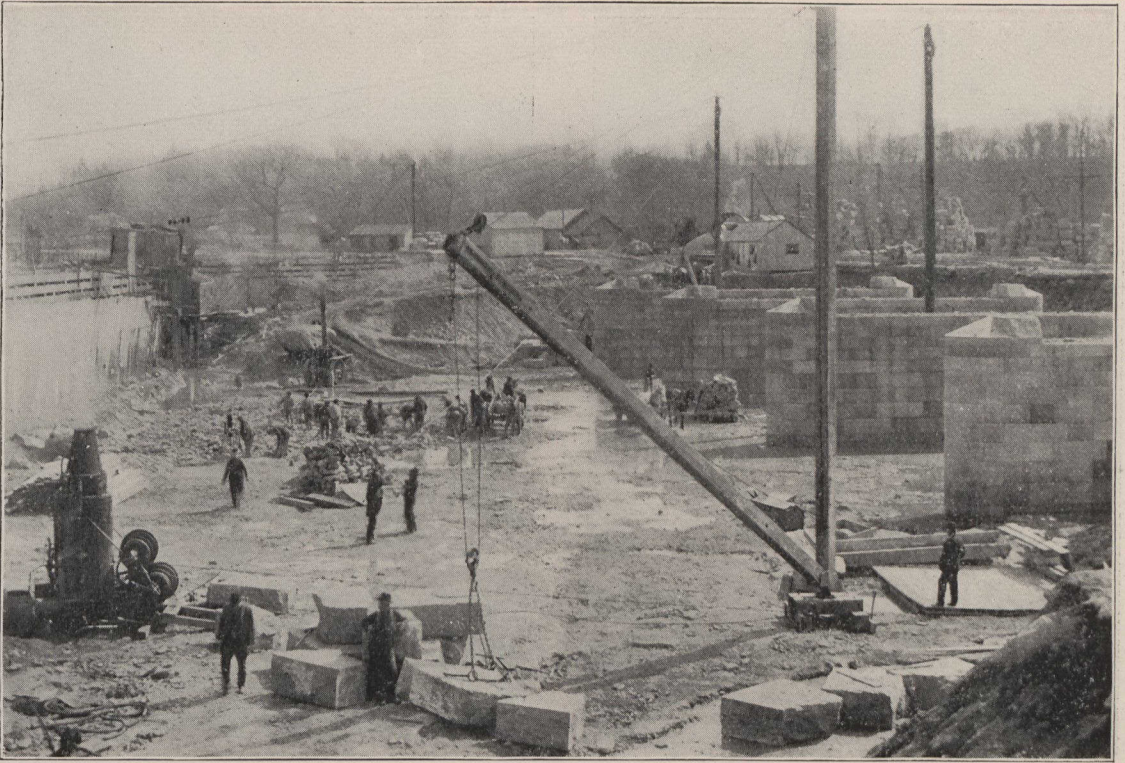
VIEW OF FOREBAY, LOOKING SOUTH
