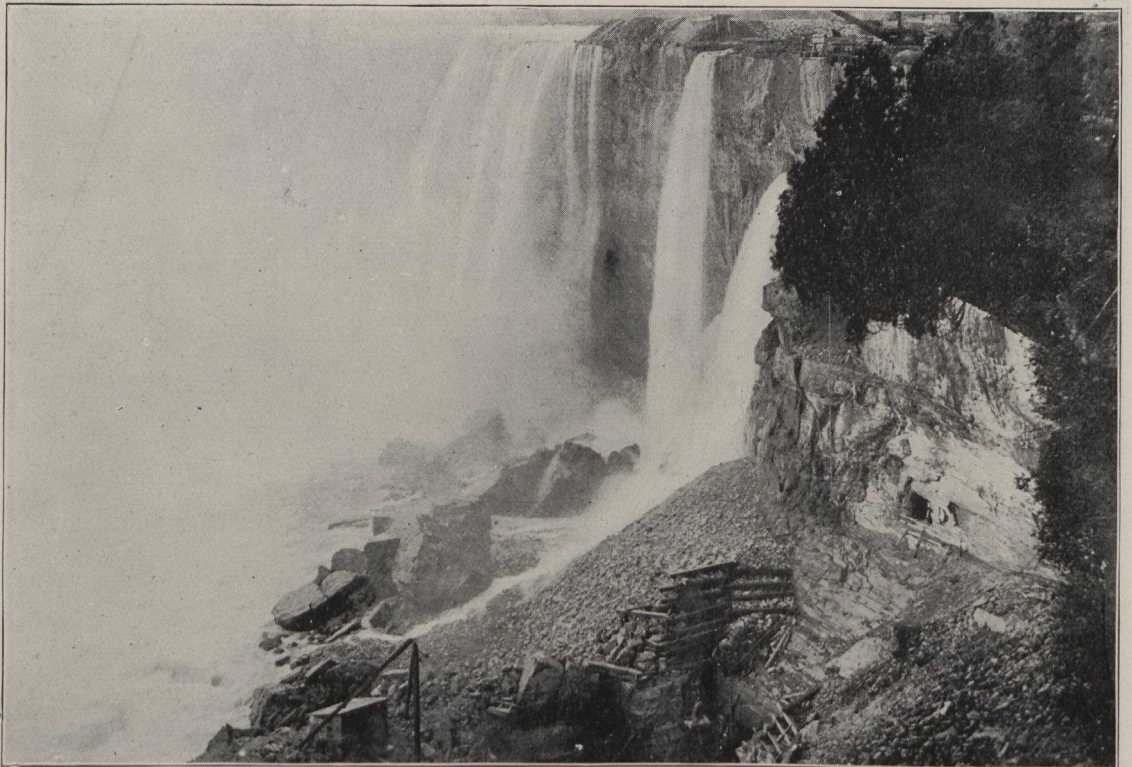
GENERAL VIEW OF PORTAL FROM TOP LANDING OF ELEVATOR
