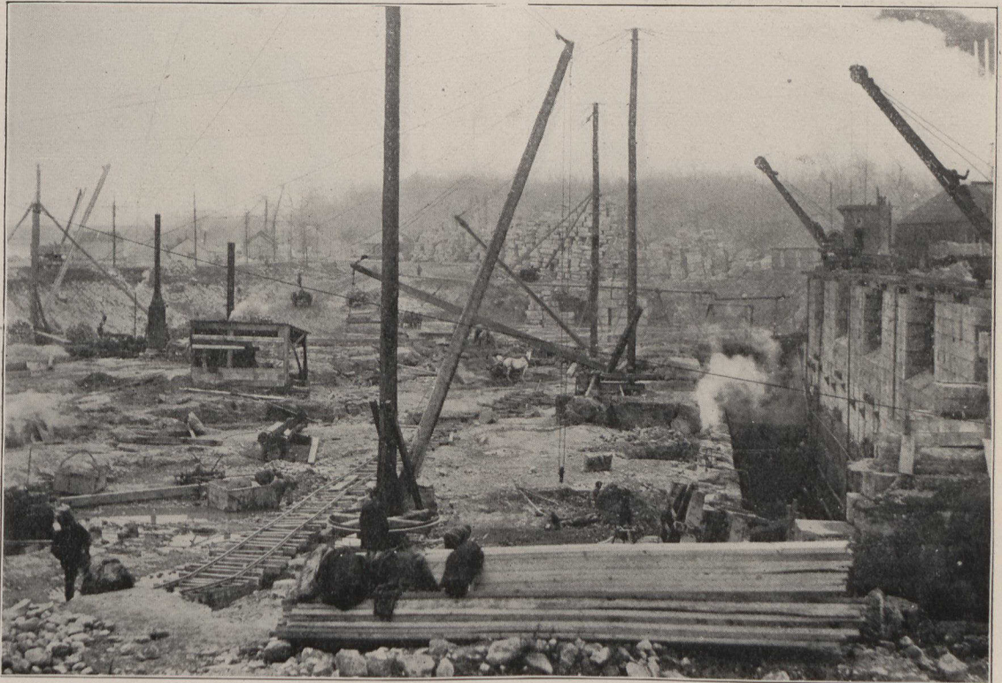
GENERAL VIEW ALONG INLETS FROM NORTH END OF PIT
