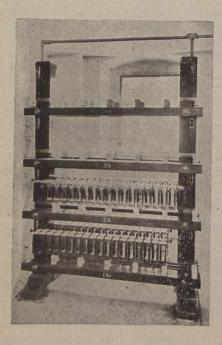
cells of storage battery, 6 ampere-hour capacity.
