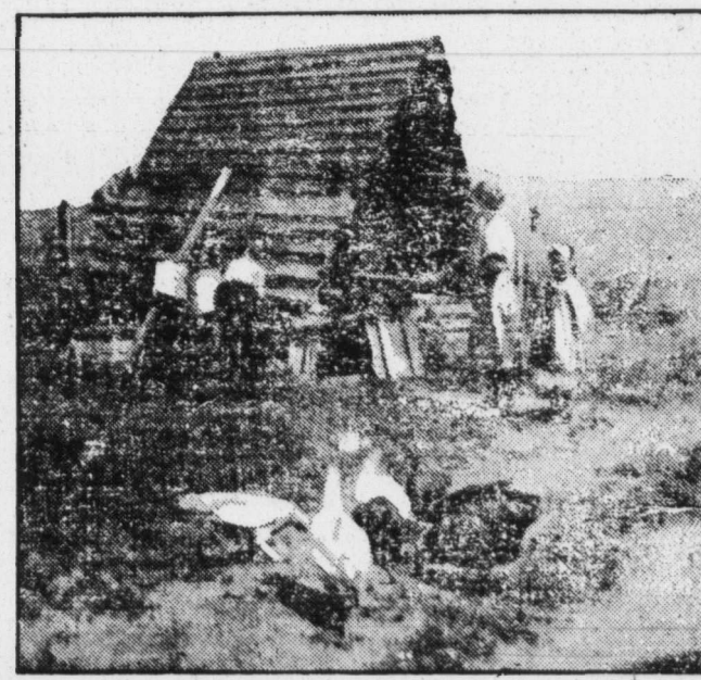
By courtesy of the C.P.R. A Quebec Roadside Oven.
