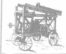
HE Neiseless Well Drilling Machine is the term usually applied to The Standard when compared to other makes, with their incessant rattle and clang. They are compactly constructed and their mechanism is built of iron and steel-not wood.
