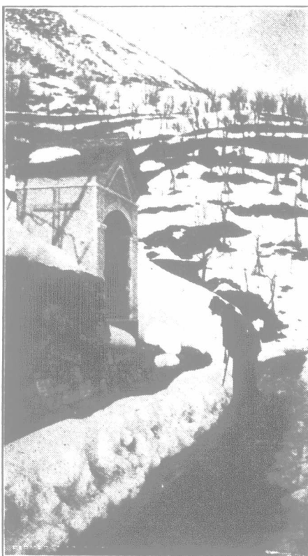
A Wayside Shrine on the Brione Road.
