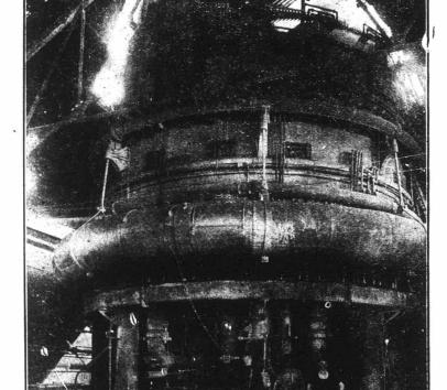
BASE OF STACK SHOWING LARGE BLAST PIPE SUPPLYING AIR TO THE TUYERES. ST.AM OPERATED MUD GUN IN FOREGROUND USED FOR PL GGING. TAP HOLE BEHIND THE MUZZLE.
