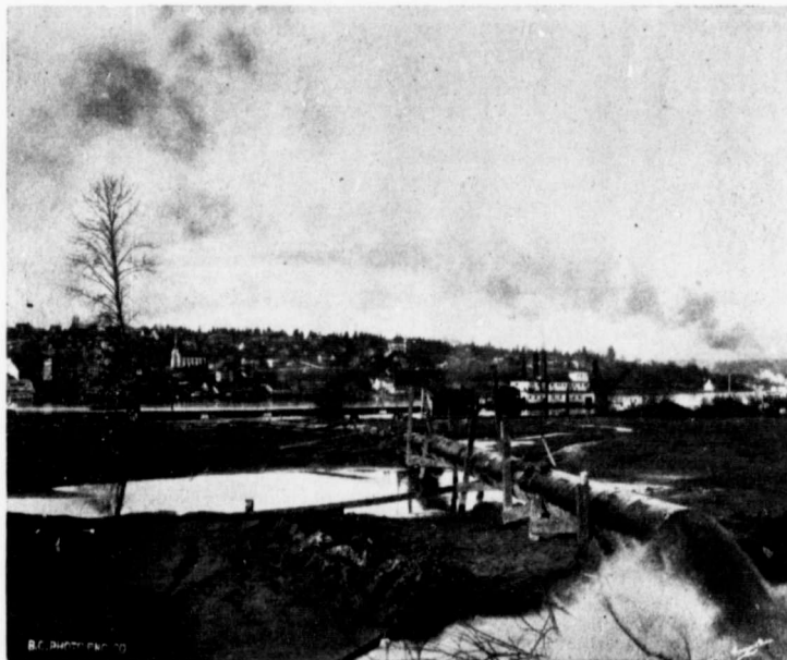
Discharge Pipe—Showing work done by the dredge at New Westminster.
