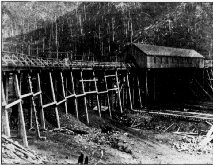
Weighing and Screening Building.
