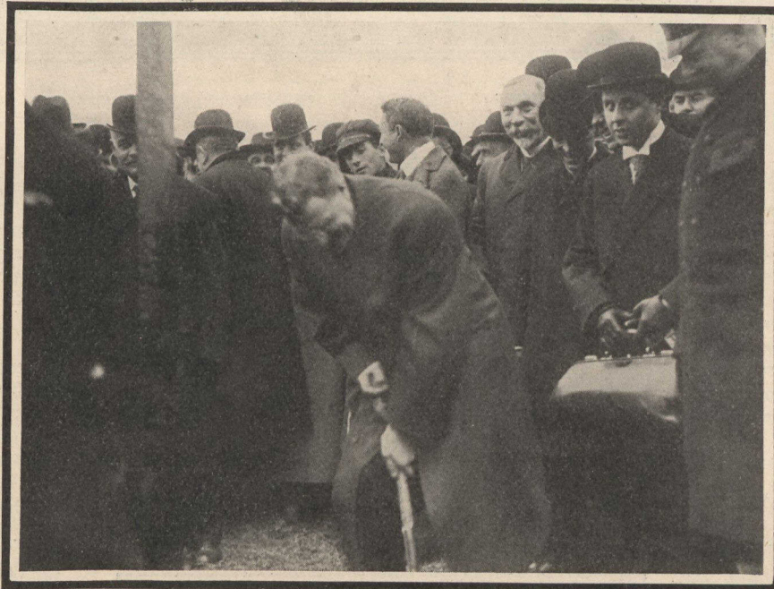
Mr. Fryer, President of the Niagara Power Union of Municipalities, turning the first sod for a power line, which is to distribute Niagara Power all through Western Ontario.
