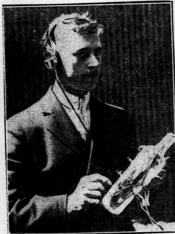
In less than seven hours Victor LaForce, C.N.R. car checker, constructed a working radio set in a bottle. He used only a pair of pliers, a screw driver and a few pieces of wire, and made all the pieces except the binding posts
