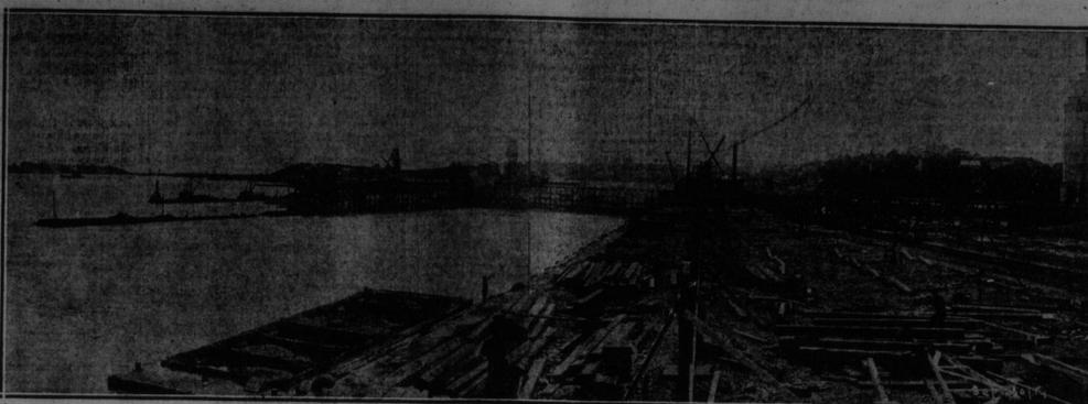
This view shows the new wharf with the uprights for the new freight shed as it appeared on September 30. Across the slip will be seen the second wharf under construction. The two huge concrete distribution towers are seen as well as one of the reclamation plants. The wharf across the slip will be completed before December.
