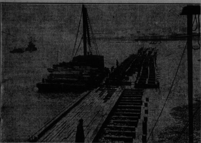
The above picture shows the cribs as they appeared on March 4, before being levelled and before any concrete superstructure had been placed in position. This picture was taken from the end of the Connolly wharf.
