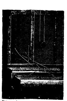
FIG. 2.—ARRANGEMENT OF SPRING JACKS, SWITCHES, AND ANNUNCIATORS ON SWITCHBOARD,
