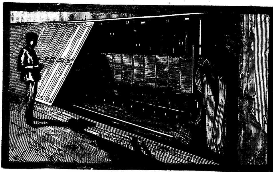
FIG. 3.—REAR VIEW OF SWITCHBOARD, SHOWING CABLES.
