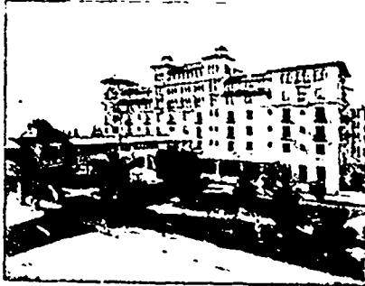
An Absolutely Fireproof Building Completed in 1893.
