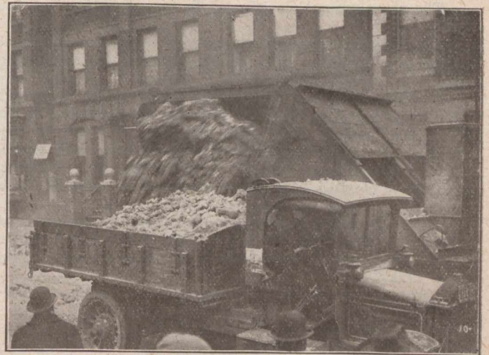
SNOW TANK DISCHARGING TO TRUCK
