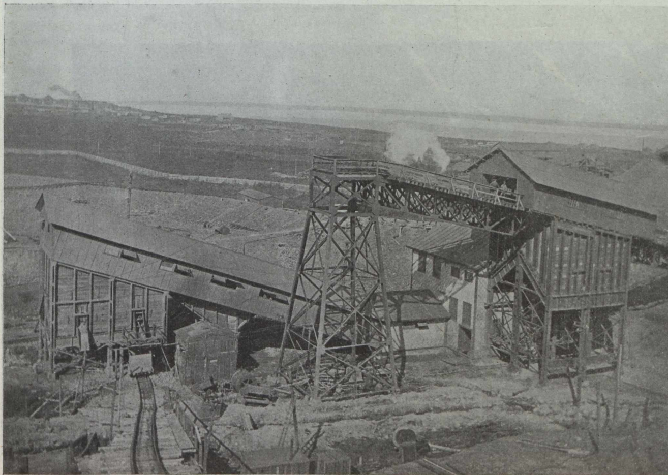
View of Dockhead, Ore Bins and Picking-Belt House at No. 3 Scotia Slopes.
