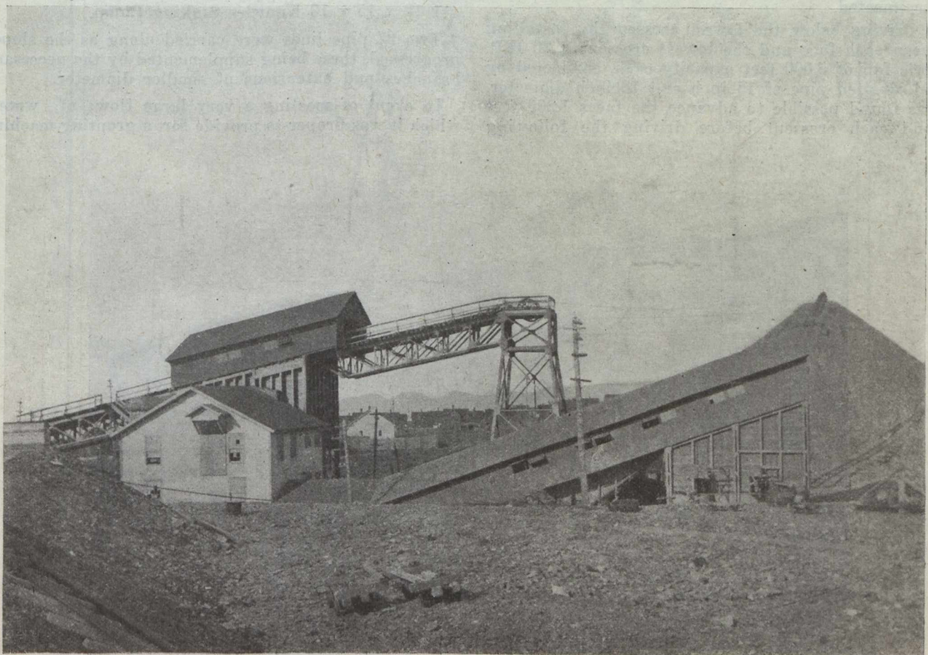
Another View of Deckhead, etc., at No. 3 Slopes.
