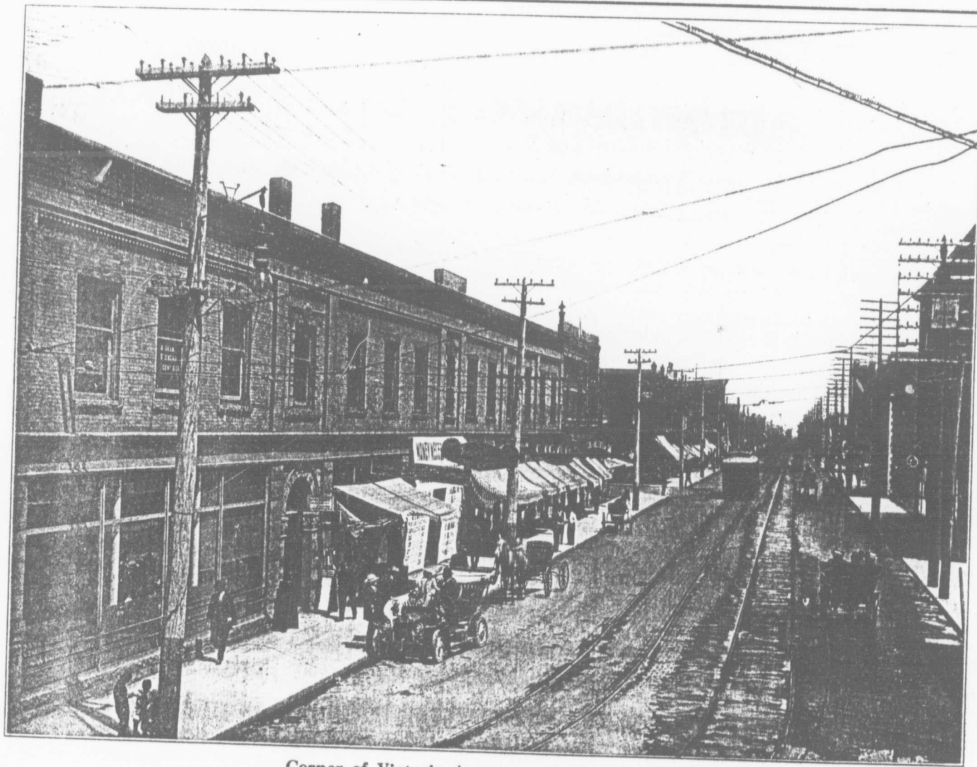
Corner of Victoria Avenue and Simpson Street
