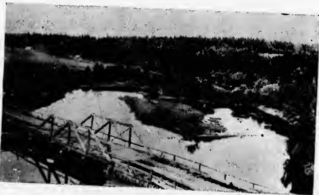
DUNK RIVER---THE BRIDGE
