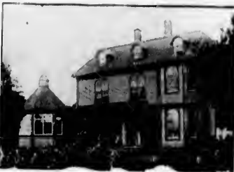
Residence of Hon. L. H. Davies
