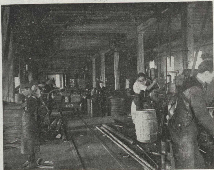
Machine Shop of the Pease Foundry Co. in Toronto; Specializing in Combination Heat and Ventilation Apparatus.
