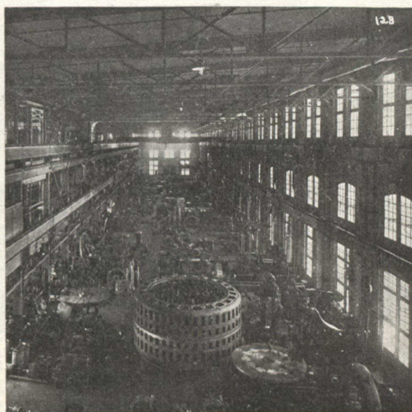
A Machinery Department in the Canadian Westinghouse Works at Hamilton, Ont. Established Under a Protective Tariff for Revenue. Output Increased 40 per cent. in 1911. Capital Over $4,000,000.
