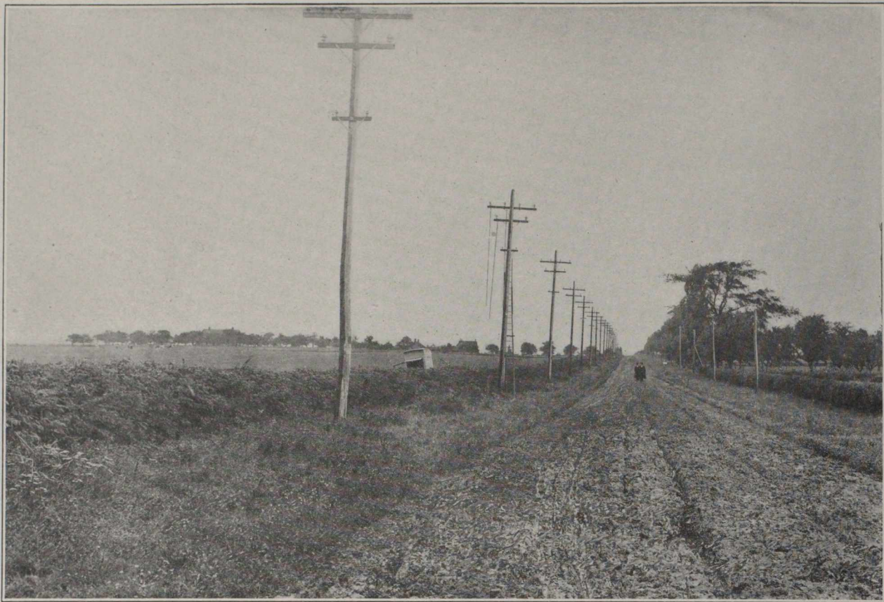
Agricultural Hydro-Power Demonstration, Aug. 28, 1912. Ontario St. looking north. Transformer wagon and connections to lines operating at 2,200 volts.
