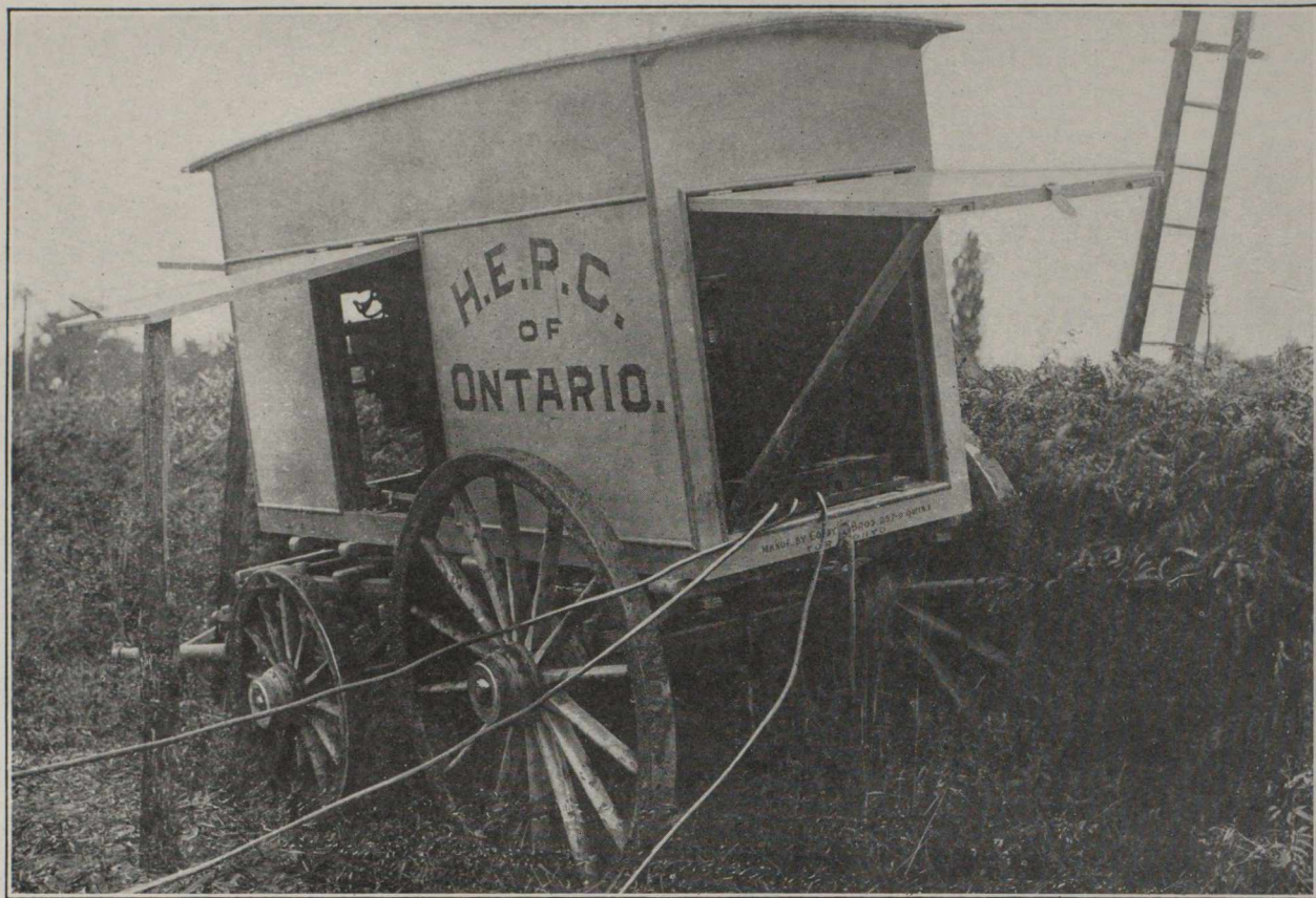
Agricultural Hydro-Power Demonstration, Aug. 28, 1912. Transformer Wagon inside hedge at Mr. Might's Farm.
