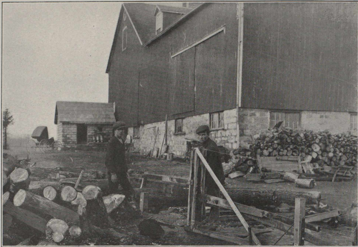
Hydro-Power Demonstration. Geo. Raymond's Farm, showing Drag Saw.
