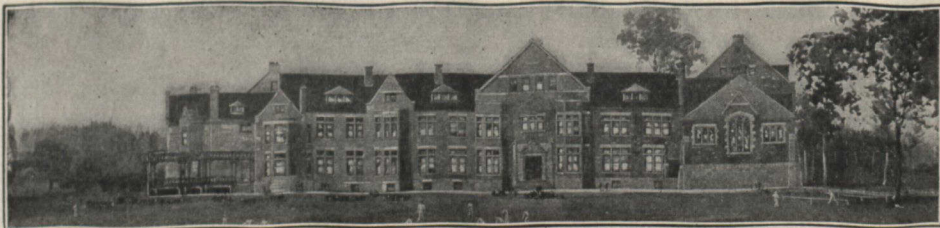
NEW BUILDINGS NOW BEING ERECTED
