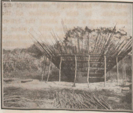
A ROOF FOR A HUT—WHEN COMPLETED, IT IS PICKED UP, TURNED OVER AND SET ON THE WALL
