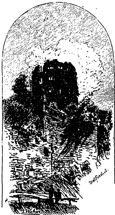
LIBRARY TOWER, HEIDELBERG.
